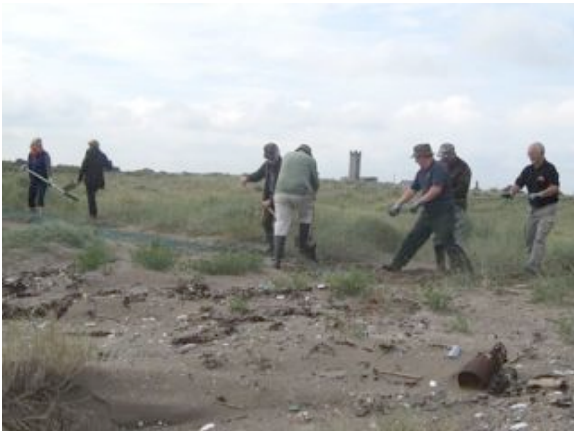
Dismantling fence Aug 2012
